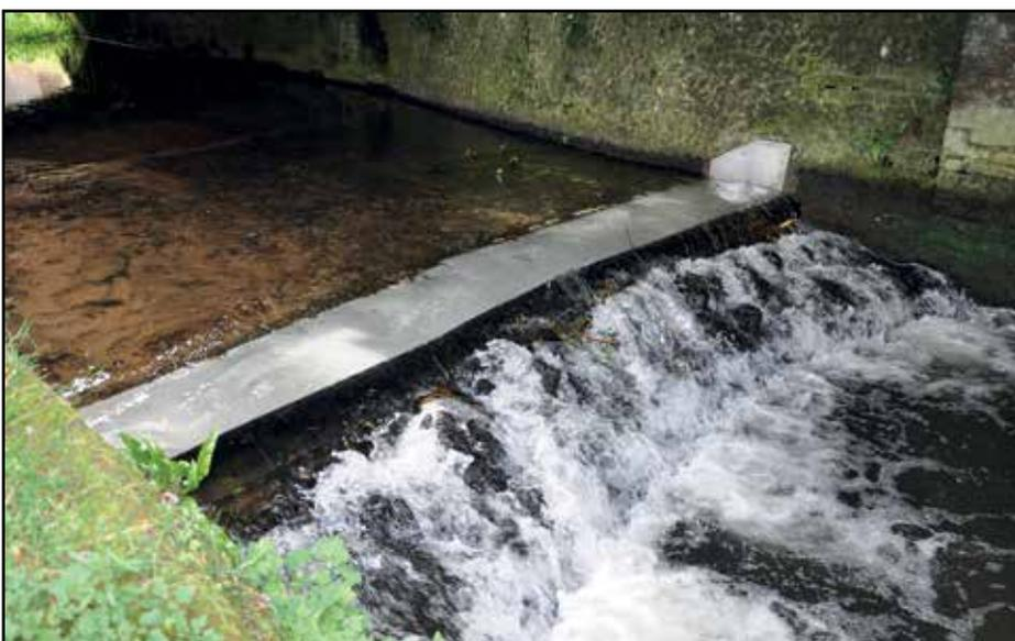
**From the top: 1. Concrete topped weir with the river flow reduced.
