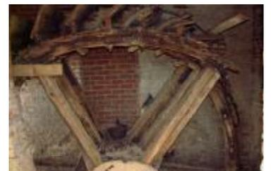
"Watermill, c. 1800, derelict at time of writing. Three storeys, brick, lucam missing. Undershot waterwheel, pitwheel and drive to three pairs of stones."
