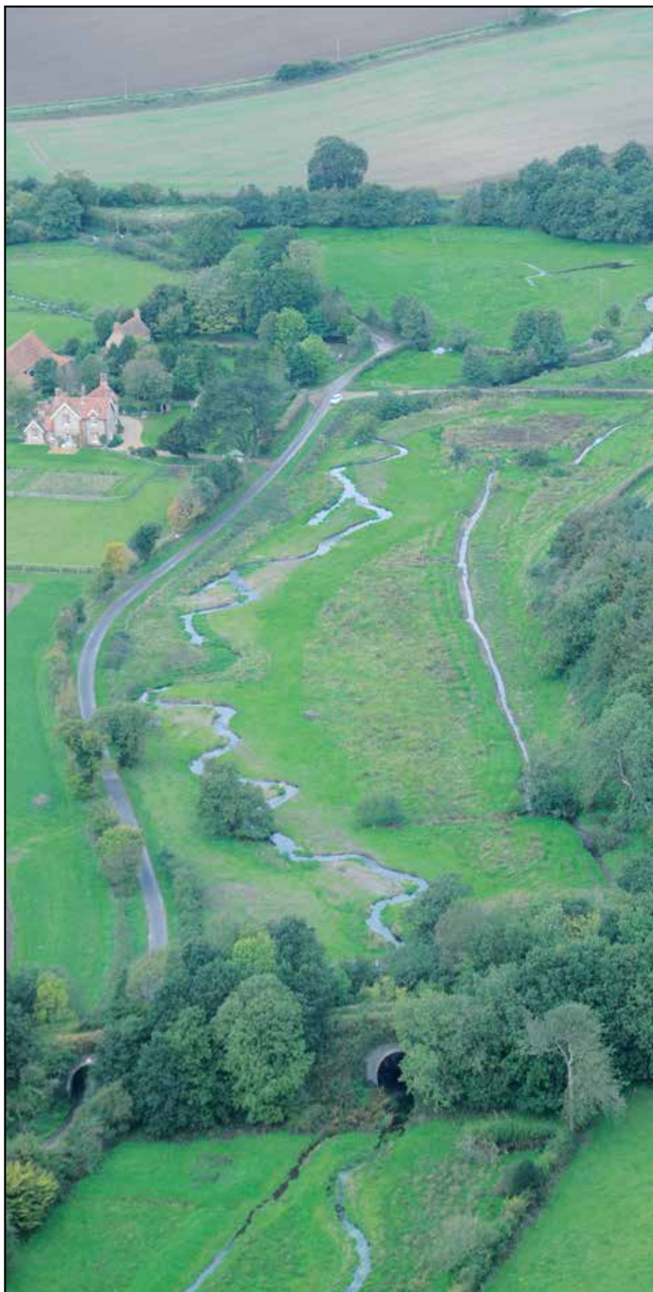
Aerial view of the completed project at 16 October 2010. The backwaters can be clearly seen. They are less visible now with the aquatic vegetation growth. The backwaters were not in the original plan. On site we realised that a complete back fill was not necessary to avoid a 'break-through' into the old channel, and was an opportunity to be taken.
