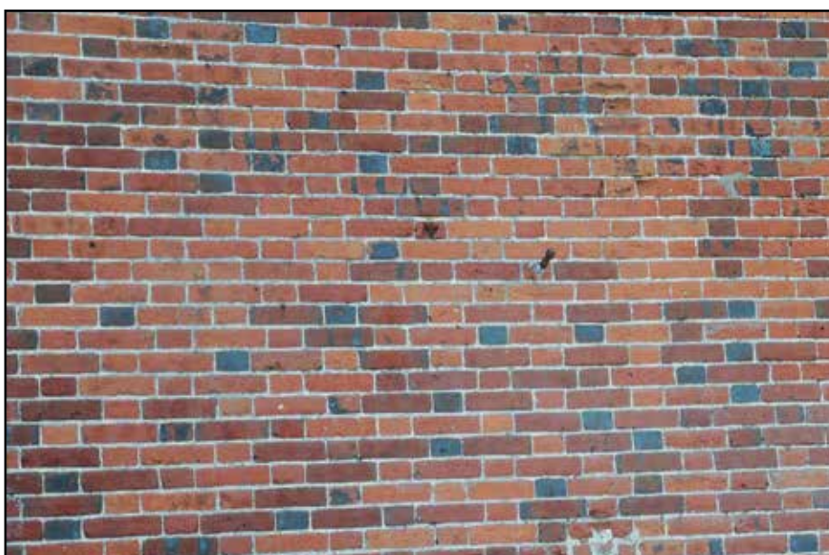
Bottom: exterior wall showing the Flemish bond brickwork.
